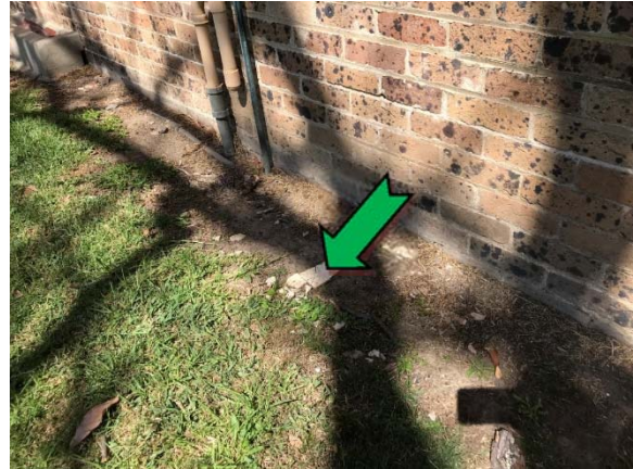
Photo 8. Exterior, south-west elevation, ground – non asbestos-containing debris.
