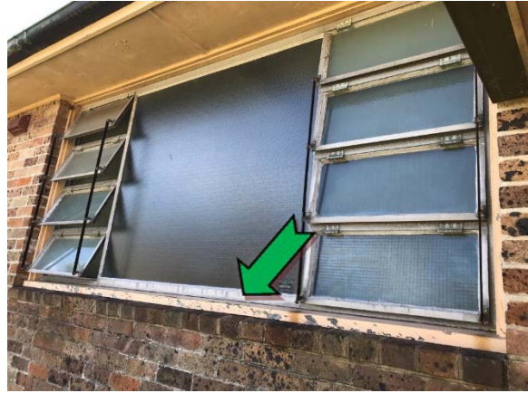
Photo 2. Exterior, metal window frames – non asbestos-containing window caulking.
