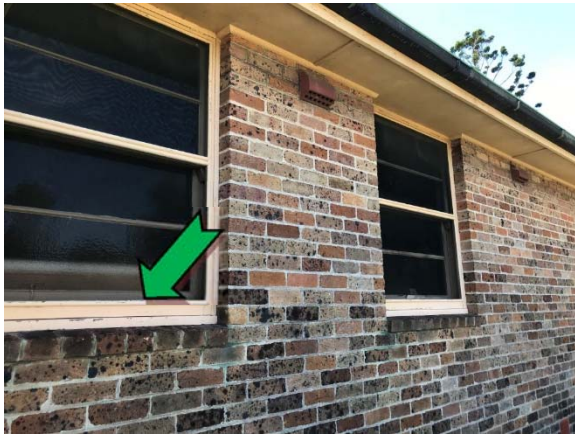
Photo 3. Exterior, timber window frames – non asbestos-containing window caulking.
